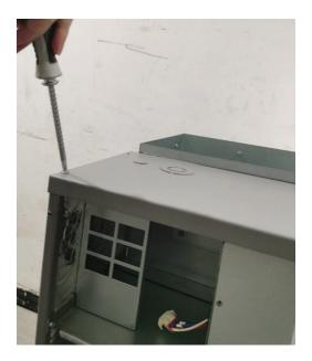
2. Remove the screws holding the electrical box in place.
