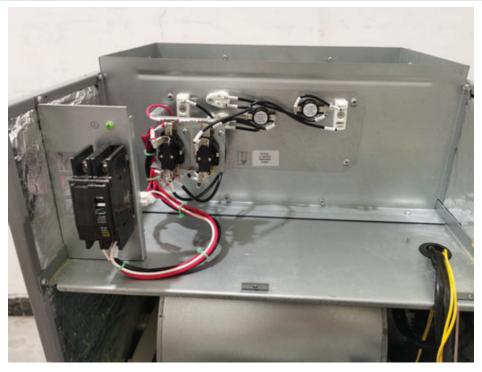
9. Once the heat kit has been properly wired, reinstall the electrical box back to its original position with the screws that were previously removed.
