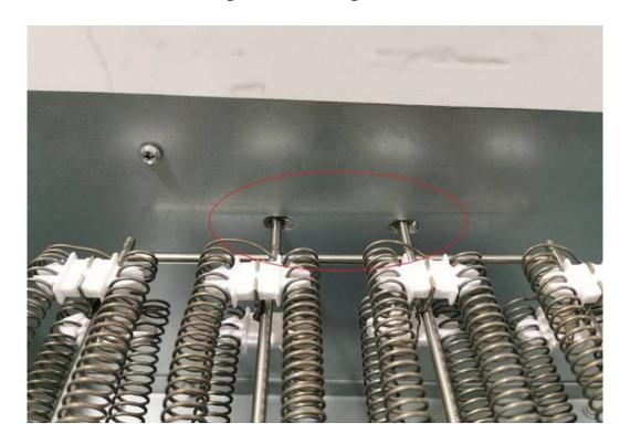
6. Secure the heat kit to the air handler by installing the mounting screws.
