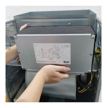
4. Remove the screws holding the access panel in place.
