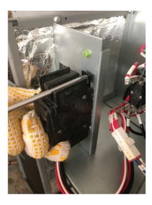
8. Connect the electric heat kit connector to the air handler wiring harness.
