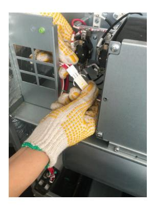
8. Once the heat kit is securely mounted, refer to the wiring diagram on the electrical box and the electrical information contained within the air handler installation manual for the proper wiring instructions and procedures.
