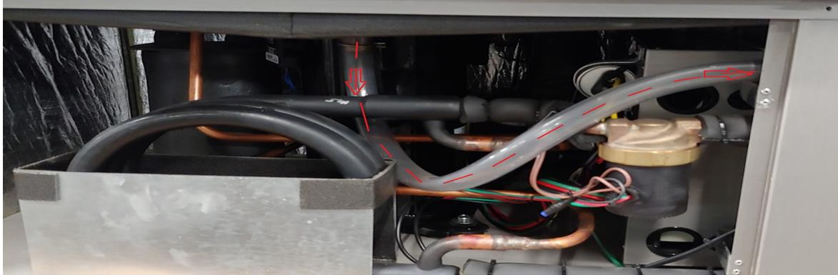
All Geocool Horizontal units are low profile. Due to this, they require **standard** P-Traps which are vented on the leaving water side and located directly **outside** the unit (see image below). Horizontal cabinets will need to be installed on a platform if not hanging in the air in order for a P-trap to be installed.
