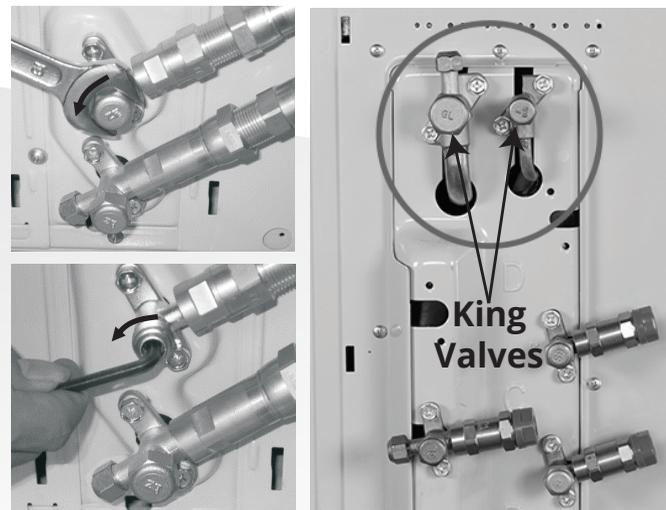
5. Using soapy water (in a spray bottle or with a brush), or leak detection spray, apply to the Quick Connect® fittings at the indoor air handlers and outdoor condenser to check for leaks. If you see bubbles begin to form, this indicates there is a leak. If so, re-tighten the connection accordingly until the bubbles are gone. Please refer to the manual for more detailed information on checking for leaks.
