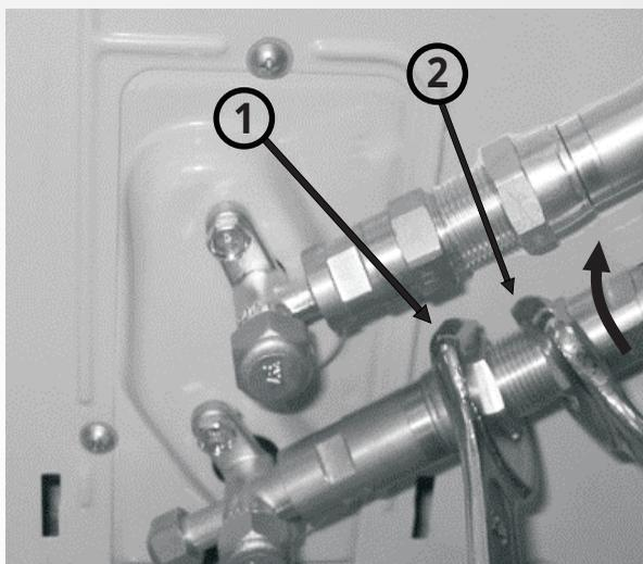
4. Then, tighten the connector slightly beyond that point to apply torque to the connector. Please refer to the manual for information about torque requirements. Repeat the same steps for the top screw connector. Now, repeat this for each air handler to be connected.
