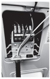
**5.** Then, you will connect the wires to the terminal block. Each wire should be numbered and correspond with a connection port on the terminal block. Match up each wire with the correct port, and firmly screw the u-lug of each wire to its corresponding terminal. Now, screw the ground wire into the bottom screw of the terminal block, as shown in the image below.
