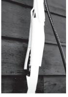
3. Now, starting at the outdoor condenser and working your way up to the wall hole, you will wrap the exposed line set and drain hose together tightly using the supplied Non-adhesive U.V. tape. The drain pipe will need to be at the bottom of the bundle (Refer to Fig. 6.3 and the image below). *DO NOT* wrap the end of the drain hose
