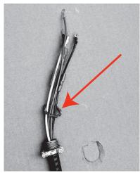
**3.** Now, pull the end of the DIYPRO™ Cable through the left hole of the outdoor condenser that was beneath the electrical cover you removed. Please refer to the image below.
