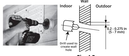
Fig. 4.3 Wall Hole Sleeve Installation
